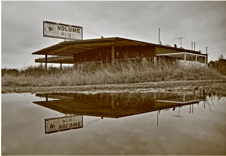
Abandoned Bill Thompson Merit
